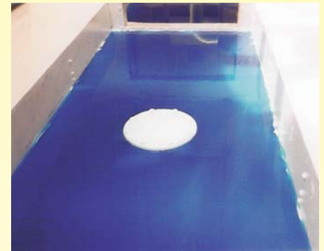
Tower basin after Pancrete XE applied
