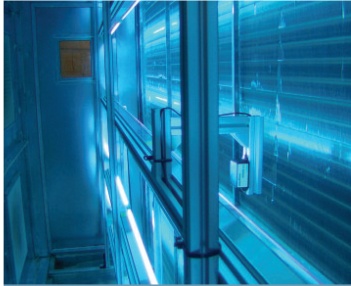
BEFORE-AND-AFTER LABORATORY CULTURES FROM HOSPITAL HVAC UNITS SHOW ANTIMICROBIAL IMPACT OF STERIL-AIRE UVGI.
